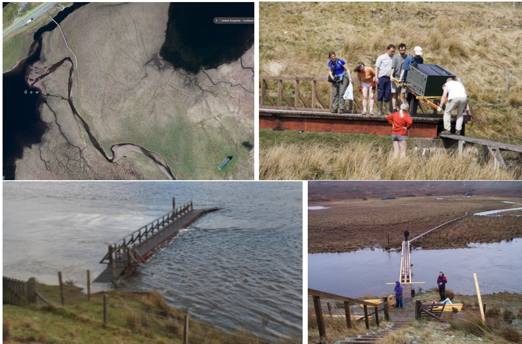
Photo 2.3: The original walkway, visible from space / in use to carry in the cooker / flooded at Christmas 2015 / and repairs underway.
